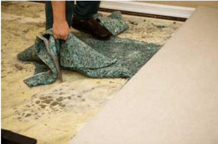
contractors remove flooring and adhesive to allow the concrete slab to cure more thoroughly. If the moisture conditions cannot be naturally remediated, installers may need to try decorative concrete, less moisture-sensitive floor coverings, breathable floor coatings, or topical moisture vapor suppression systems. If moisture has caused severe damage, the whole floor (concrete and covering) may need to be reinstalled.
