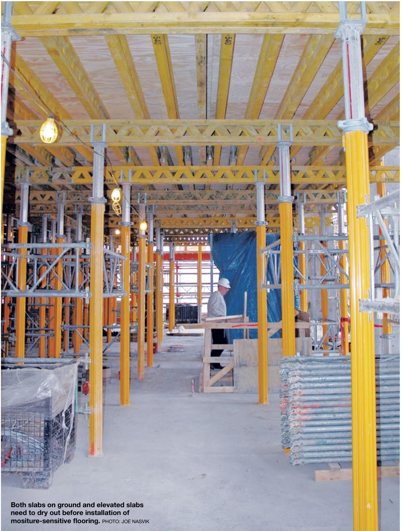
**Both slabs on ground and elevated slabs need to dry out before installation of moisture-sensitive flooring.** PHOTO: JOE NASVIK
