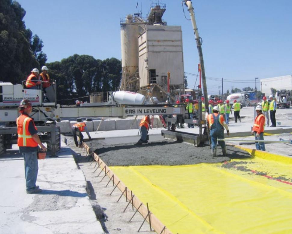
**This self-dessicating concrete exterior placement was made on a vapor barrier to prevent the very low water content from being sucked up by the subgrade.** PHOTO: U.S. CONCRETE
