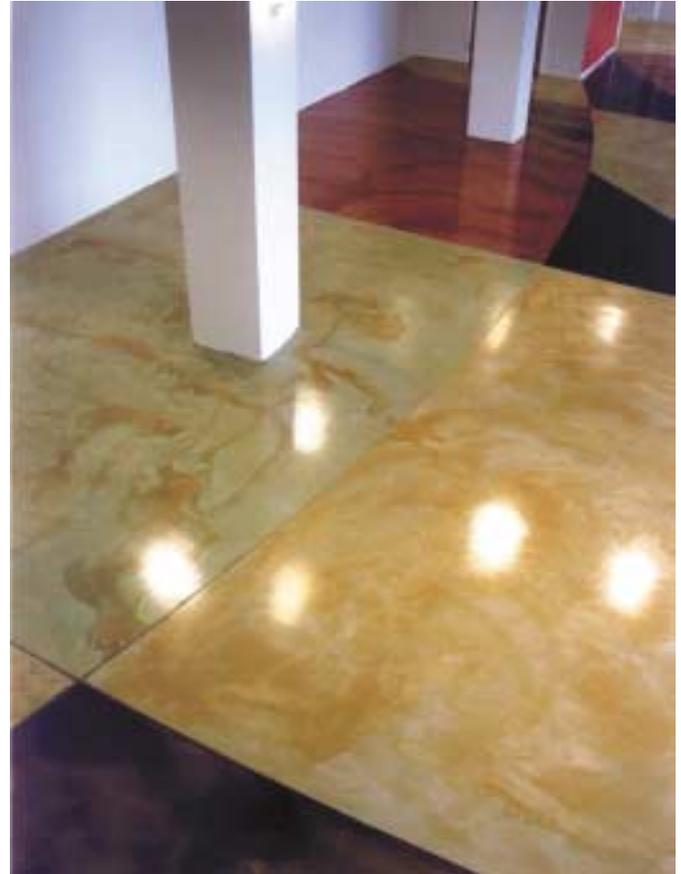
Fig. 7: Stained cementitious overlays provide a durable, decorative surface for concrete slabs on and above grade. They allow the designer and owner almost unlimited options as to patterns and colors (photo courtesy of Ardex, Inc.)
