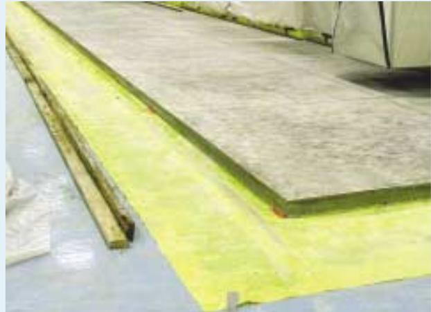
If an existing slab was built with no vapor retarder beneath it, a new slab, placed over a vapor retarder, is one renovation option
