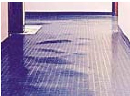
Fig. 1: Many flooring failures result when high moisture levels and a high pH beneath low-permeability floor coverings combine to produce adhesive failure
